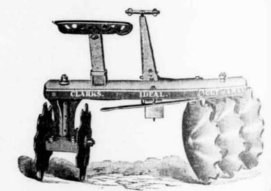
I am showing you a cut here of Clark's Cutaway Plow combined, worked by two borses, which leaves your land thorough and turned to the depth of 7 to 9 inches. The recent packing rain the land to break cloddy with the usual plow, but this tool leaves the Corn Planter. To see it work is to appreciate it. I sold 25 of the North Carolina last year as a test and every one is giving entire salish.
