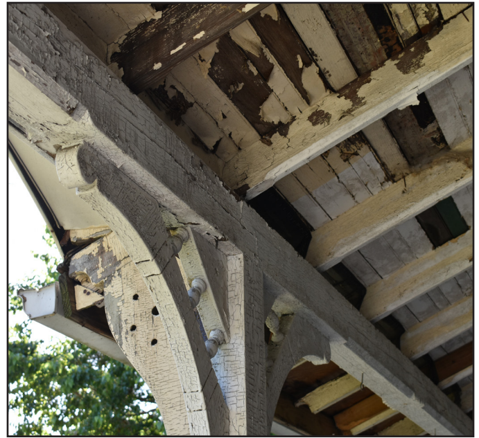
Figure 9: Cracking and flaking paint, like the paint seen on this porch, can expose wooden detailing to moisture and dirt, promoting further damage. Be sure to monitor the condition of the paint on Carpenter Gothic features and clean regularly.
