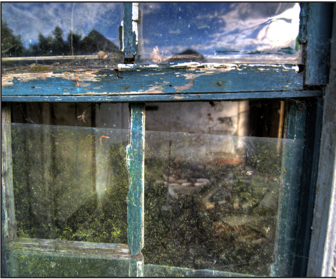
Figure 8: Though possibly not as severe as the window of this vacant house, lack of routine care can allow for moisture to penetrate wooden architectural details and cause extensive damage.
