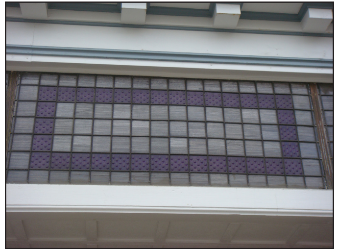
Fig. 7: South Elm Street, Greensboro, North Carolina. Detailed photograph of a prismatic glass transom utilizing different colors and textures.
