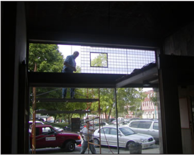
Fig. 10: Restoration of the Opera House's prismatic glass transoms. Courtesy Delphi Preservation Society, Delphi, Indiana.
